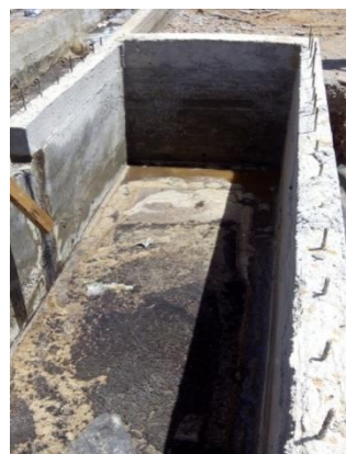
Figure 2. Photography of leachate collection basin
