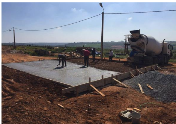
Figure 1. Photography of platform under construction
